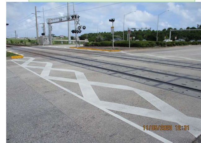
Linton Blvd and SFRTA Rail as installed by FDOT.
